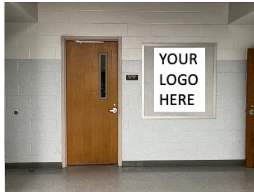
Next to Tech. Ed. IPC & Doors to Classrooms
